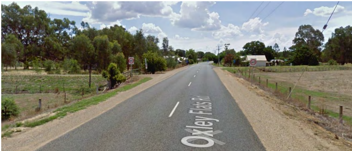
Figure 12-26 Trafficable road crossing (raised road) in Wangaratta
