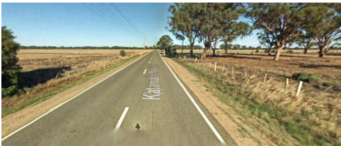
Figure 12-31 Approximate location of eastern floodway on Katamatite-Nathalia Road approximately 400 metres east of Kinnairds Road looking east (Google 2017)
