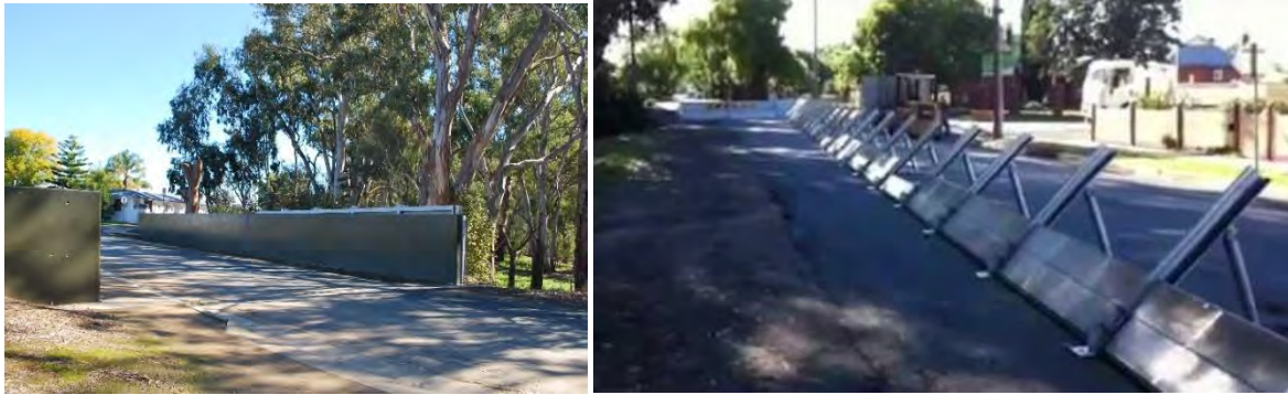
Figure 12-27 Examples of temporary flood gates and demountable walls in Deniliquin, NSW and Nathalia, VIC
