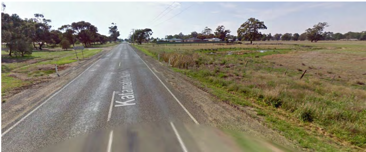
Figure 12-30 Approximate location of western floodway on Katamatite-Nathalia Road at lower end of hospital depression looking east (Google 2017)
